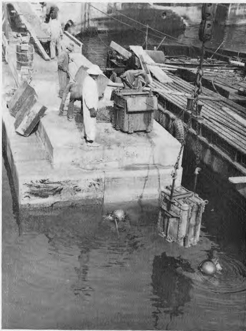
Lowering concrete container
