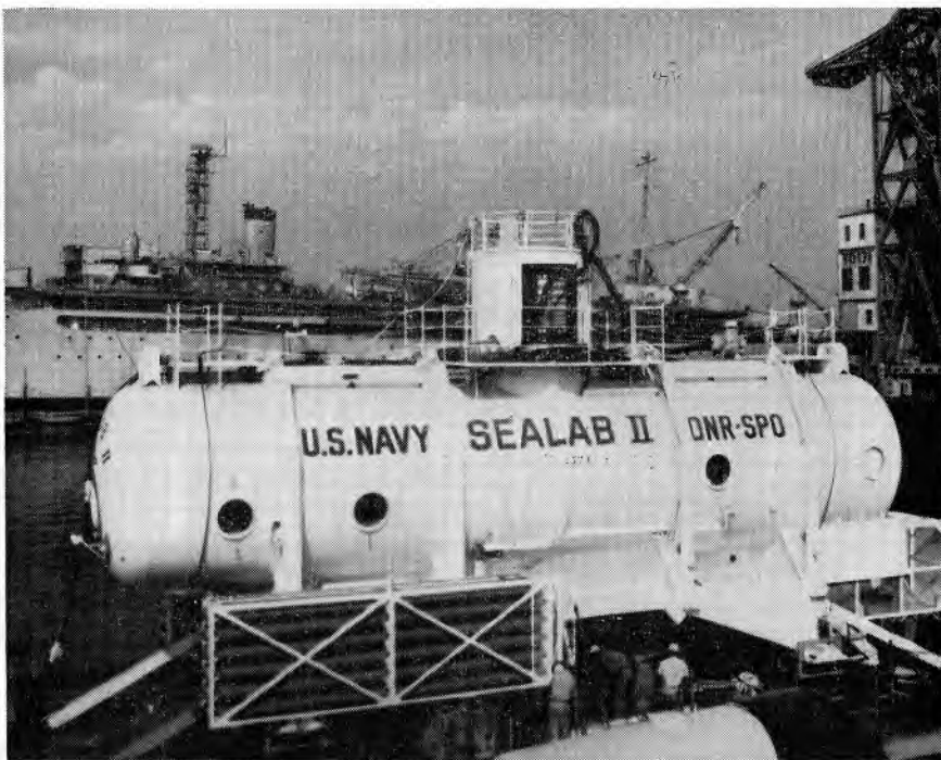
SEALAB II on barge at the Long Beach Naval Shipyard shortly before being put in the water for towing to La Jolla, California, and stationed 210 feet below the ocean's surface.
