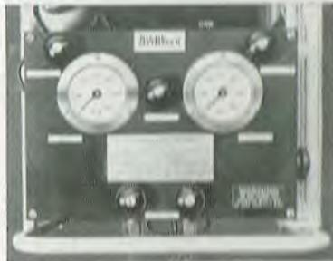
filter and control panel is mounted in a tubular steel carrying frame and weighs approximately 400 lb. It can be used independently or incorporated in a static installation.
