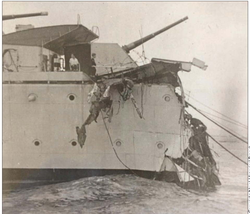
Figure 1 - HMS Volage, her bow blown off by a newly laid mine - 22 October 1946.
