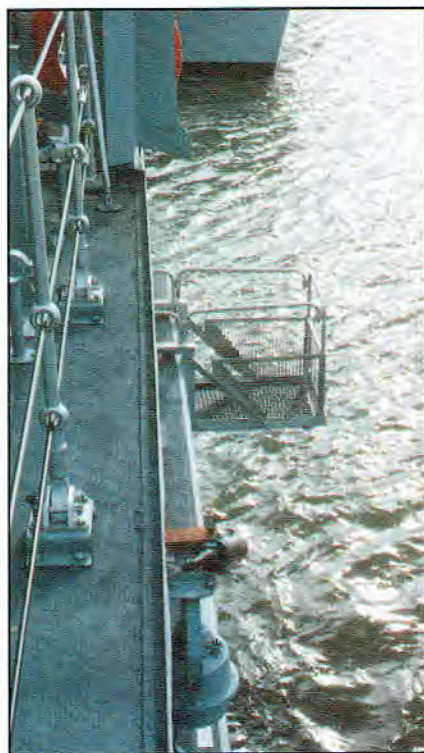
Port quarter view of 'Hero' platform
