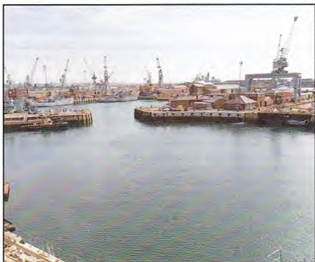
● The view looking northwards across 2 Basin. At left is HMS HUMBER, a River Class MSF of MCM10, in the background are three Ton Class MHC's of MCM 3 and an Oberon Class submarine is docked down in Number 11 Dock at right.
