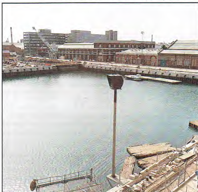
● View of the south-east corner of Number 2 Basin, with a Ton Class Minehunter refitting in Number 8 Dock and contractors working on the jetty improvements. In the foreground, atop the lamp-post, is one of the new transit beacons to aid safe entry through the narrow entrance to the Basin.
